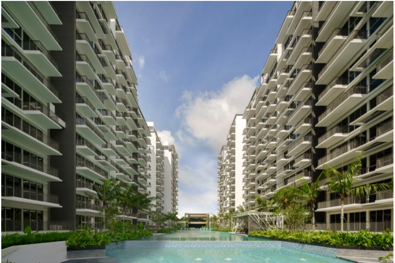
Front view of CityLife@Tampines, which was awarded TOP on February 3, 2016
